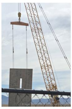
Conceptualized in the 1900's a tilt-up method of construction utilizes large concrete panels cast onsite and then raised into position with a crane. Here, walls are lifted at Array Technologies' new facility.
