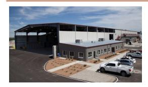
FRIEDMAN RECYCLING CENTER Building Size: 87,000 square feet Services Provided: Design-Assist-Build, Site Work, Concrete & Rough Carpentry Klinger built this pre-engineered metal building for Friedmam to provide recycling for the City of Albuquerque.
